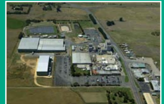
MCS Facility, 5331 Great Ocean Rd, Allansford
